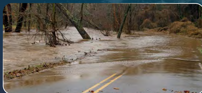
Flooding caused by heavy rains
