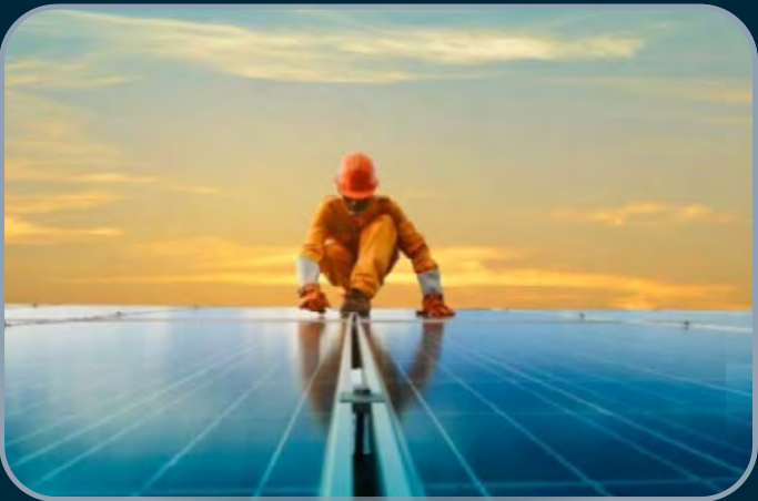
Photovoltaic installation maintenance
