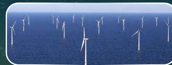
The 160MW Horns Rev (Horns Reef) offshore wind farm in Denmark
